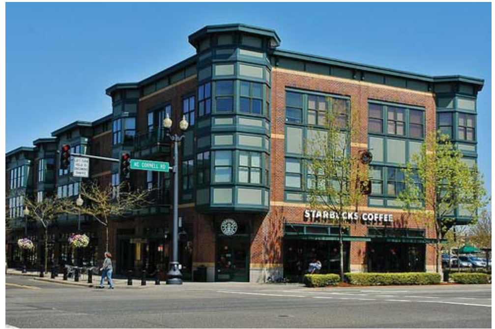
Example of residential lofts over retail in a downtown setting
