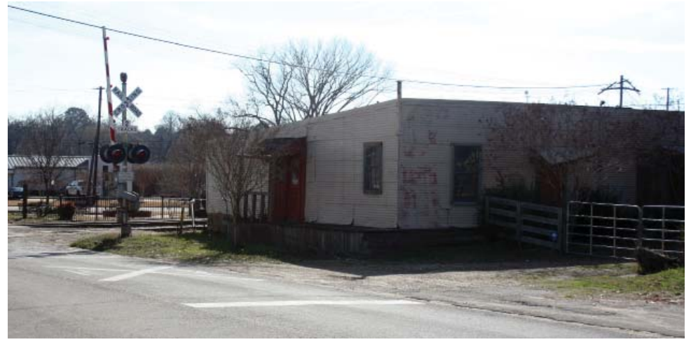
Vacant building along the west side of N. Pinkerton Street
