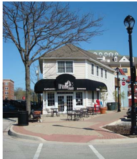
Revitalized buildings provide opportunities for shops and cafes
