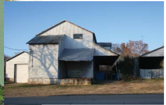
Neglected barns present opportunities for demolition and redevelopment
