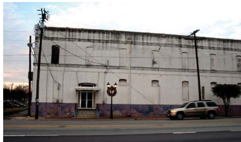
Restore window openings and repair/replace with historically appropriate window designs
