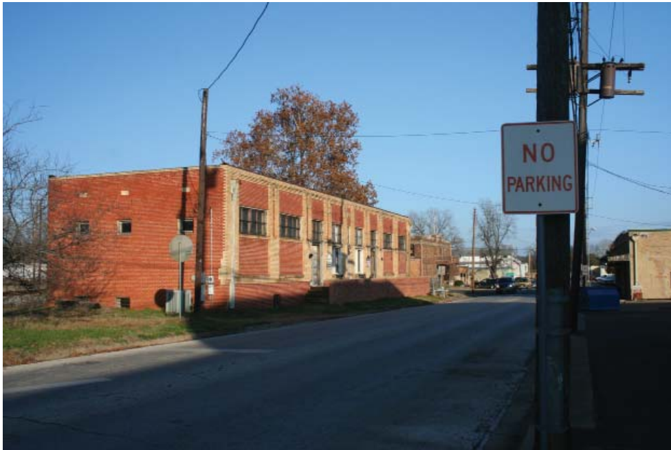
E. Larkin Street - north side needs landscaping and enhancements to building
