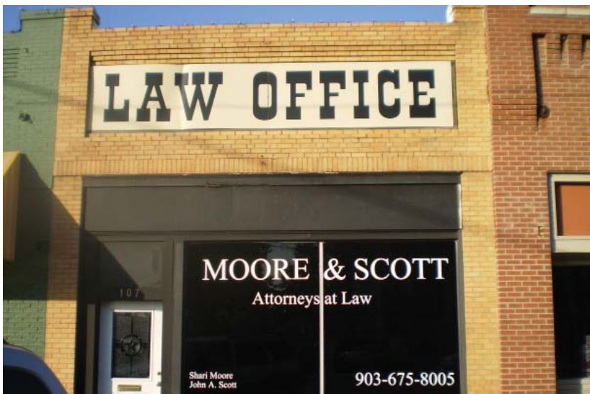
Signage dominates façade and windows
