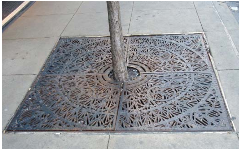
Routine care and maintenance of tree grates and street trees contributes to a safe and inviting pedestrian environment
