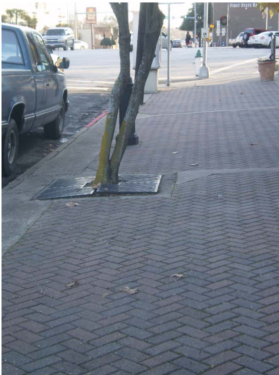
Existing vegetation has outgrown tree grate, creating ADA accessibility hazard
