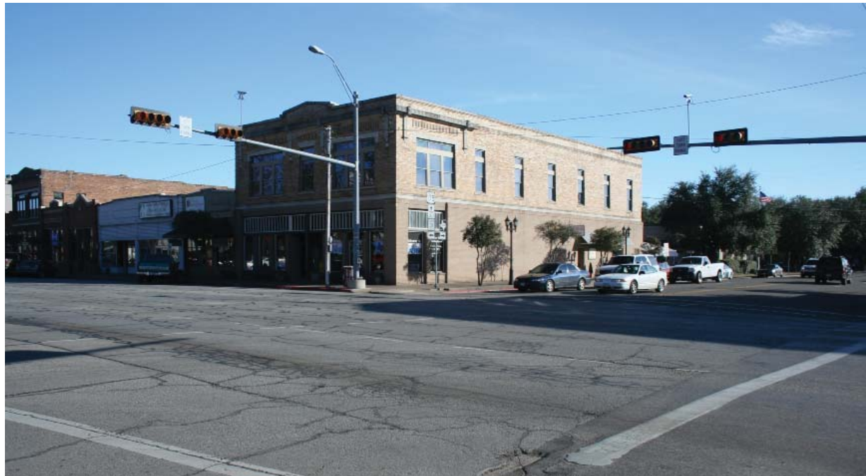
Pedestrian crossings around the square create safety and distance concerns
