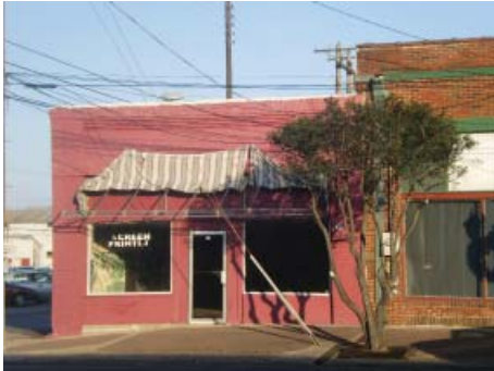
Dilapidated façade and landscape
