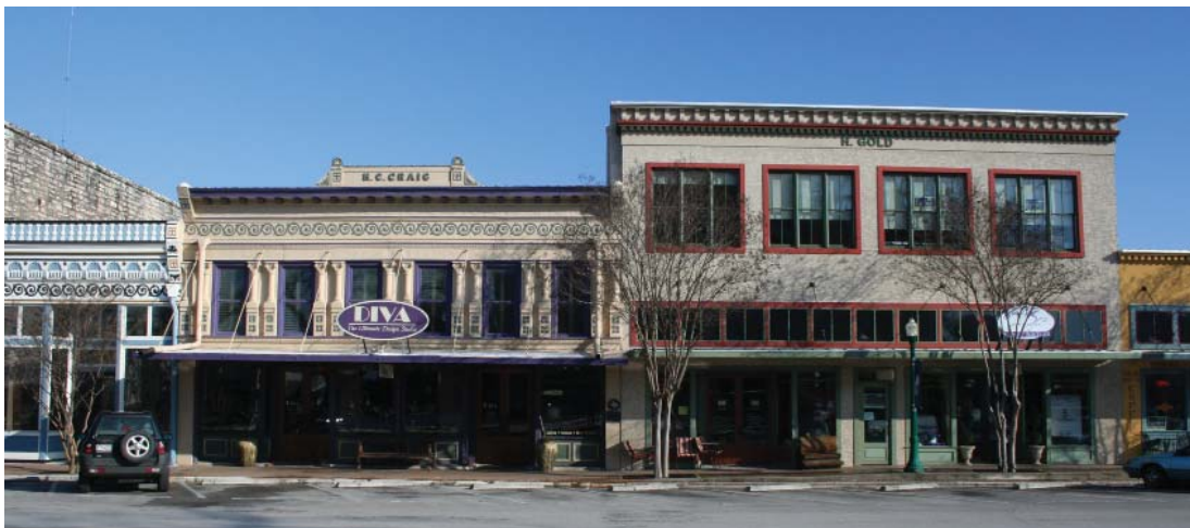
Mixed use buildings with active street scene
