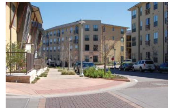
Colorful pavers, crosswalks, lighting and landscape all contribute to a pedestrian friendly environment
