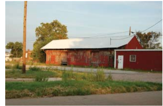
Vacant feed building
