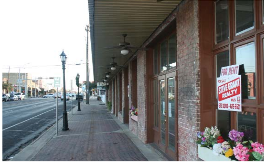
Several buildings have been rehabilitated and are ready for occupancy
