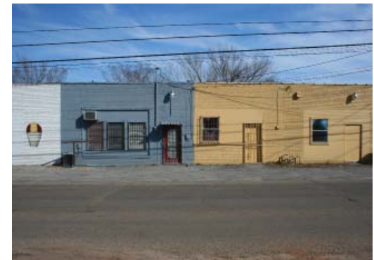
The area on N. Pinkerton needs sidewalks and landscape as well as its facade rehabilitated
