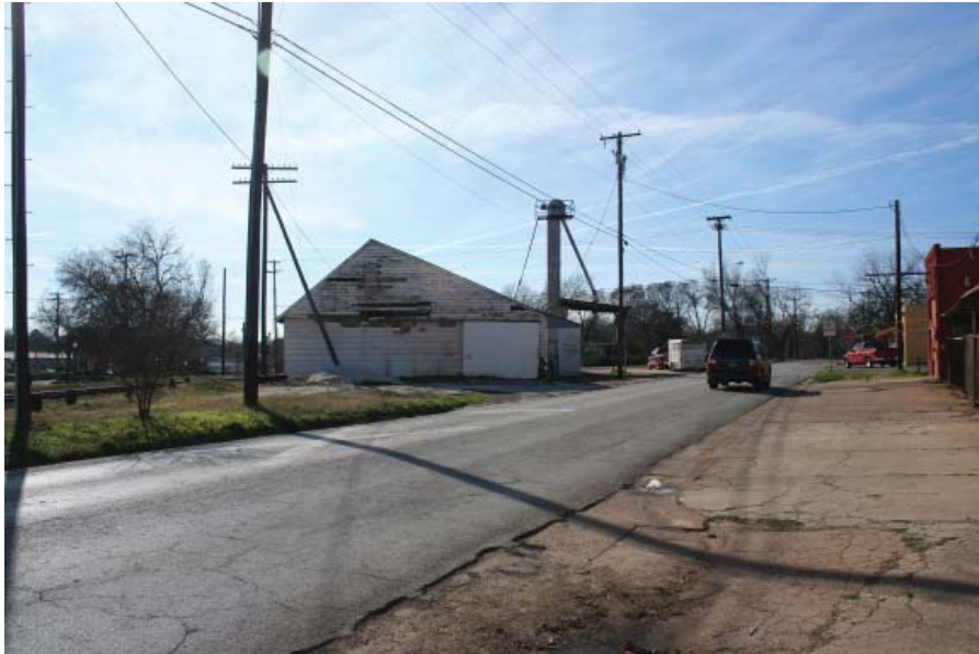
E. Larkin Street - Building is dilapidated and could be removed
