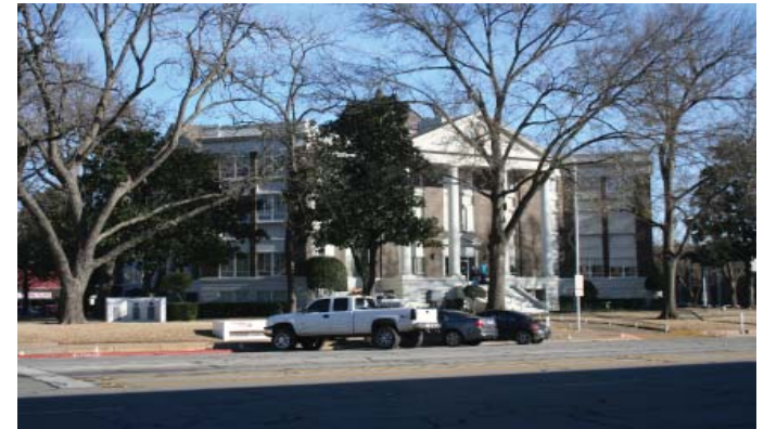
Henderson County Courthouse
