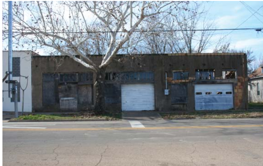
This building is a prime candidate for tear down and redevelopment
