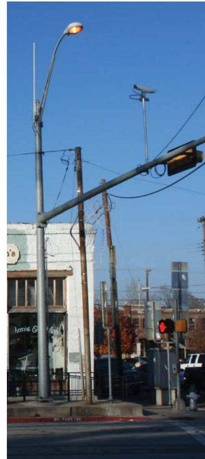
Current galvanized cobra lights and signal poles could be upgraded or enhanced
