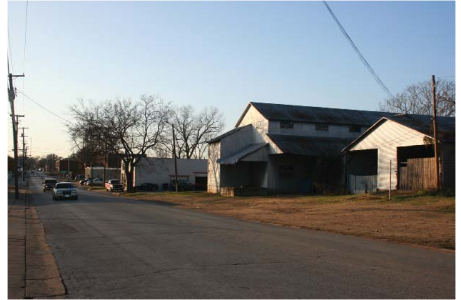
East Larkin Street - Warehouses and barns detract from downtown environment
