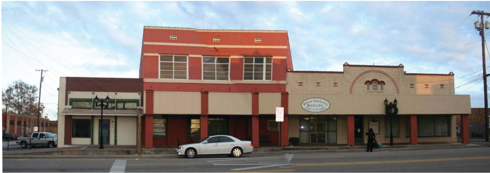
Opportunities exist to restore buildings to their historical appearance through appropriate window spacing, trim and double hung windows
