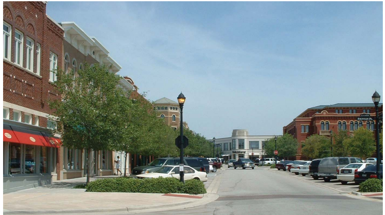
Buried power lines contribute to a more inviting streetscape
