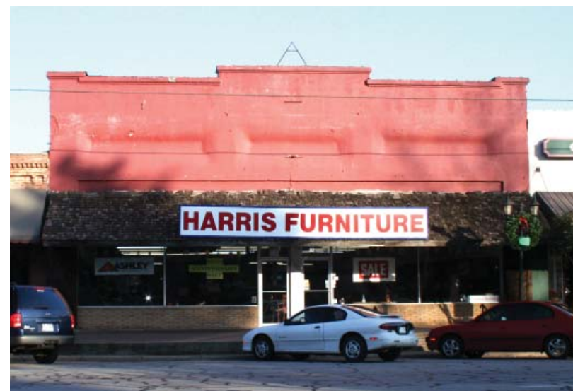
Restore original second story façade materials and design elements and replace awning and sign with designs that complement the building's architectural character
