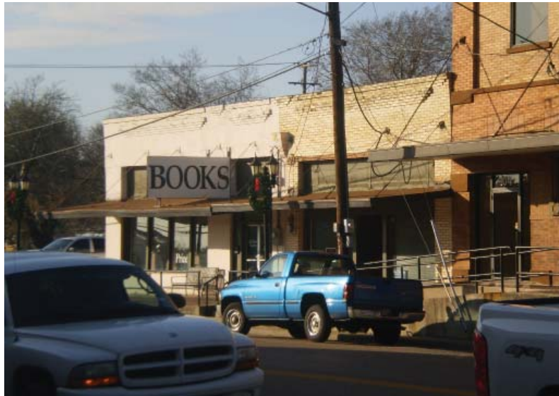
Electrical wires clutter building façades
