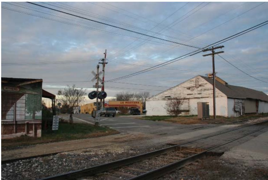
East Larkin Street - Opportunity for redevelopment
