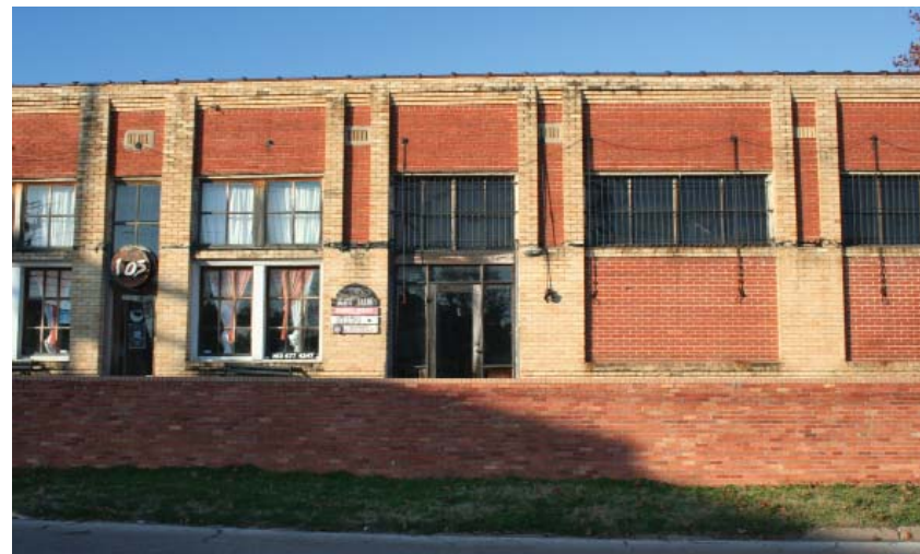
Remove security grilles from windows to reveal the building's character
