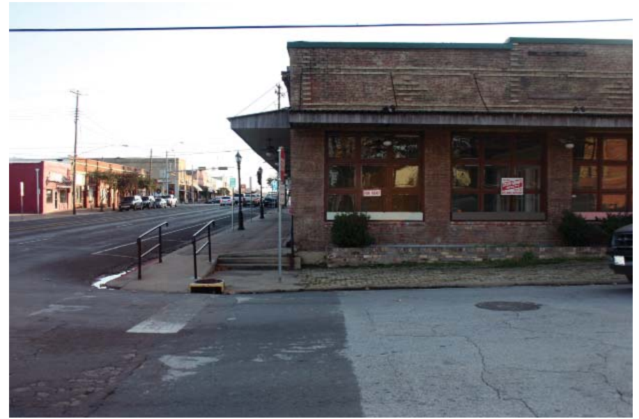
E. Larkin Street - Northwest corner at N. Palestine has potential for establishing a pedestrian friendly environment through the integration of crosswalk pavers, site furnishings and landscape
