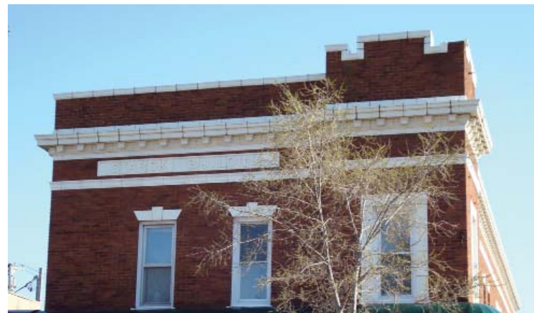
Parapet walls enhance the visual appeal of historic buildings
