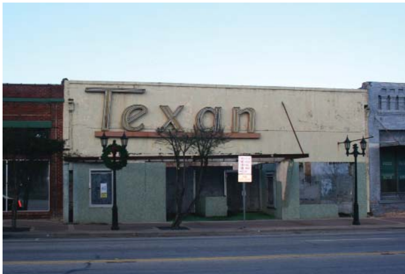
Dilapidated façades negatively impact the streetscape
