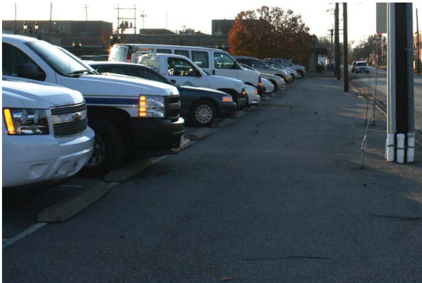
E. Larkin Street - North edge of public parking lot needs a landscape buffer to soften its appearance and a defined walkway for pedestrian traffic
