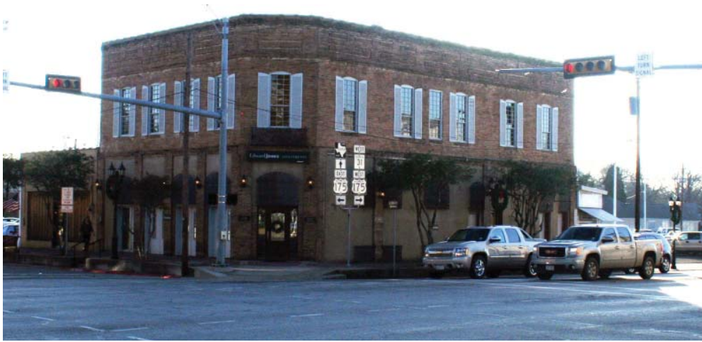
Southwest corner of Corsicana Street and Prairieville Street
