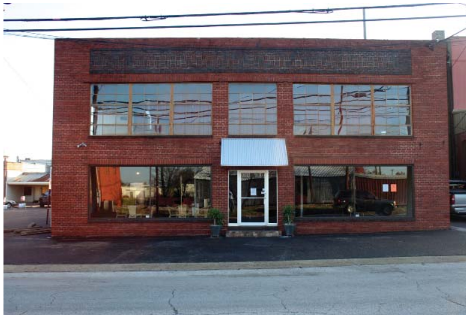
East Larkin Street - Restored historic building demonstrates potential for creating an attractive downtown environment, although still lacking landscape and furnishings
